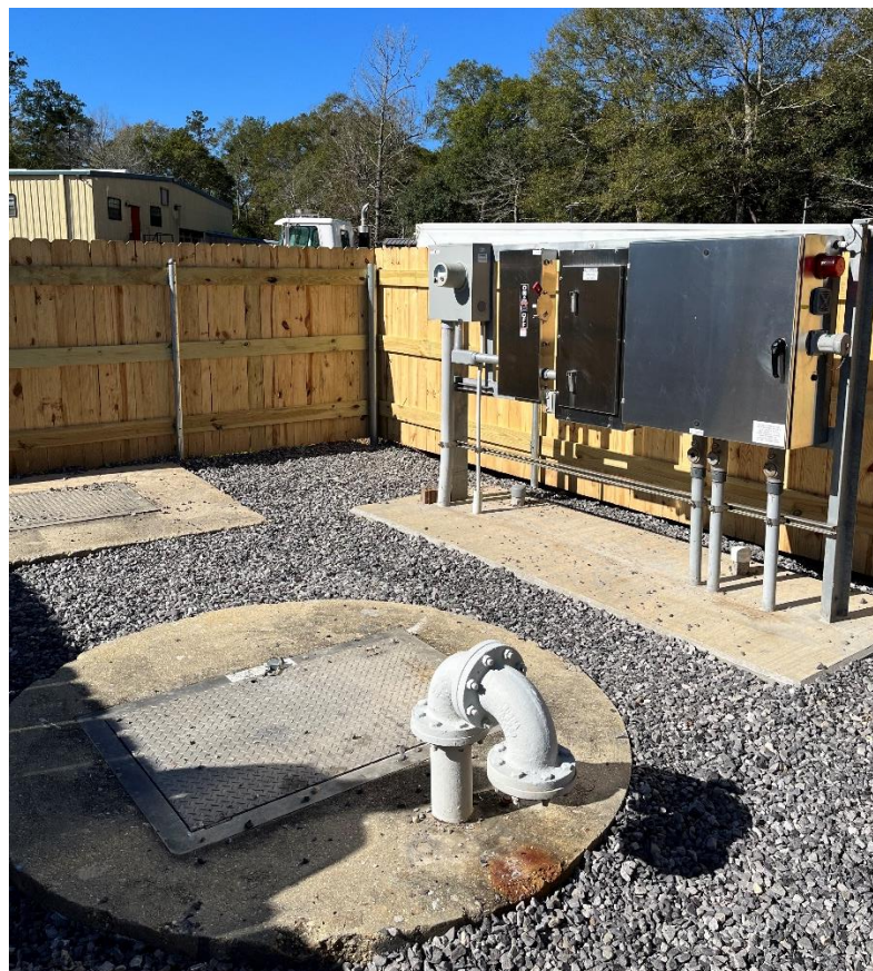
Picture 4: Lift Station Rehabilitation; new control panel
