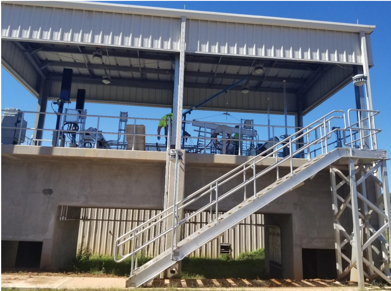
Picture 1 – New UV structure at WWTP
