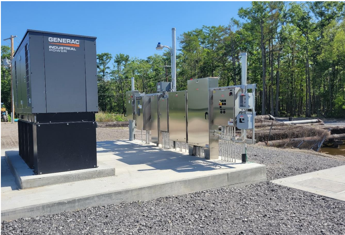
Picture 4: WWTP Rehabilitation; new generator & electrical controls
