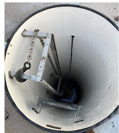
Picture 3: new manhole fiberglass lining
