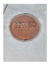
Picture 1: New Sewer Manhole with new ring & cover along concrete roadway
