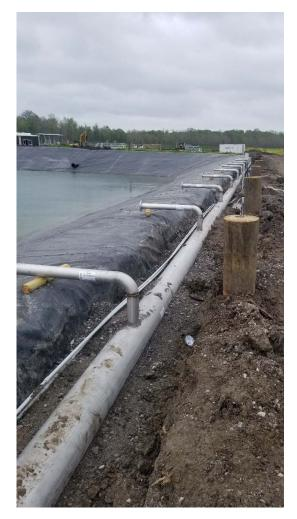
Picture 1: WWTP earthen aeration basin with liner and aeration piping
