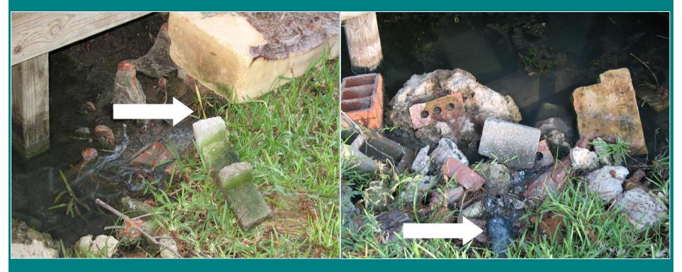
The failing septic system was also discharging directly into Cross Lake.
