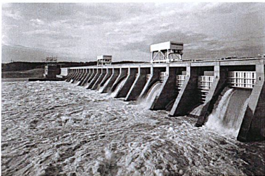
Pickwick Landing Dam on the Tennessee River, Hardin County, Tennessee, 1939. Photo by the Tennessee Valley Authority (K-1850, flickr, Creative Commons Attribution 2.0 Generic license, image resized) .
