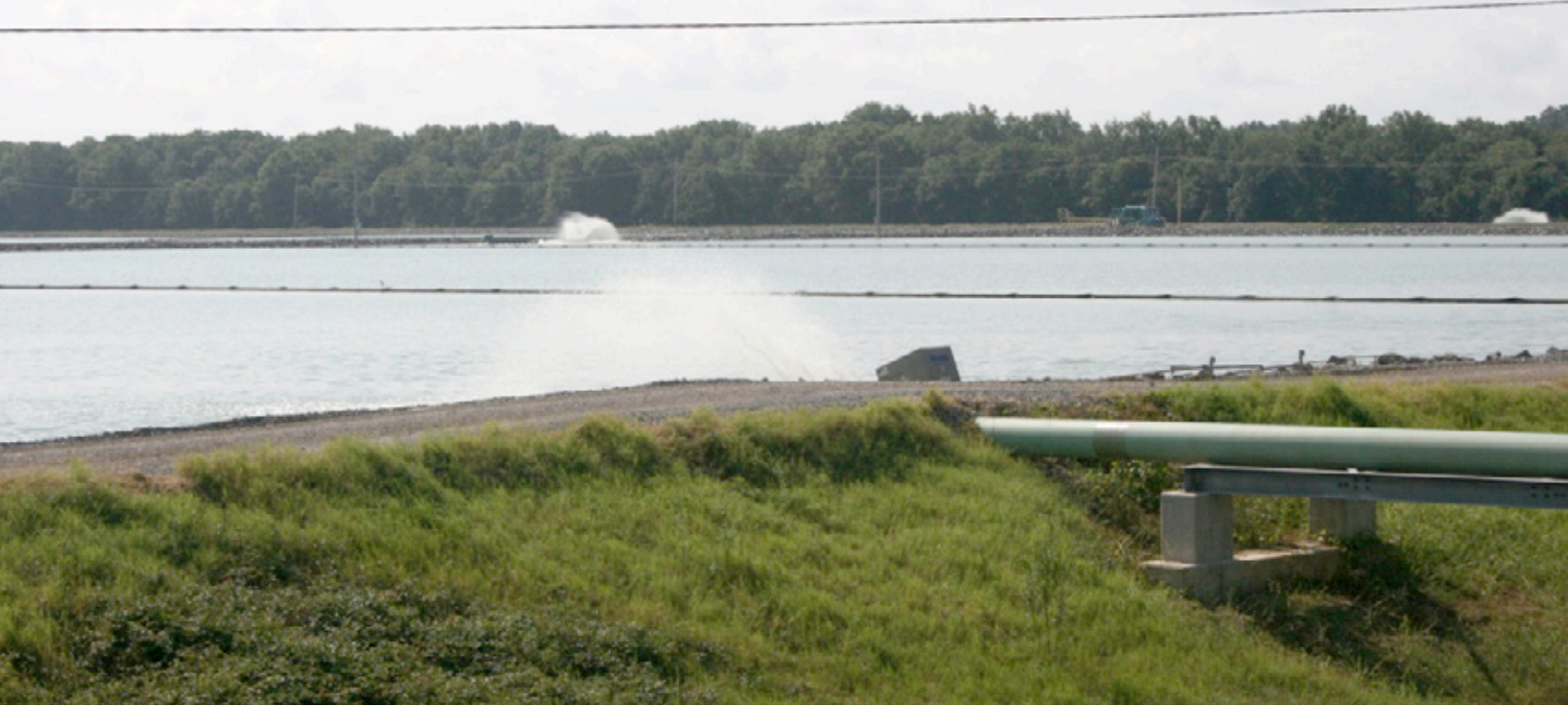
Aerators at the Sparta Re-use facility spray water into the air as part of the treatment process.
