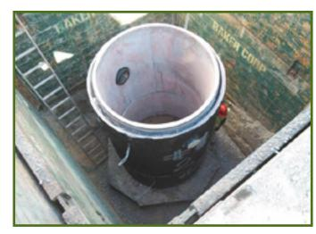
A wet well under construction at the Mansura project.
