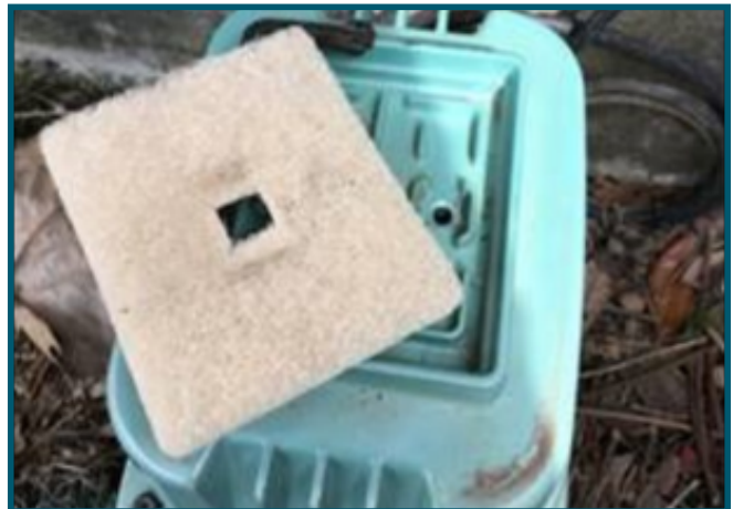
Figure 6. Cleaning/replacing air filter on the aerator is part of the outreach education program
