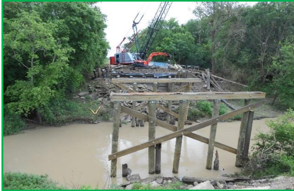
Figure 20 Replacement of the Bridge at site 4C in Bayou Chene
